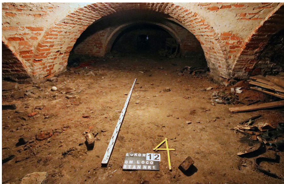
Fig. 3. Łuków, Łuków district, lubelskie voivodeship. View of the crypt before the cleaning works were carried out (photo by J. Michalik)
