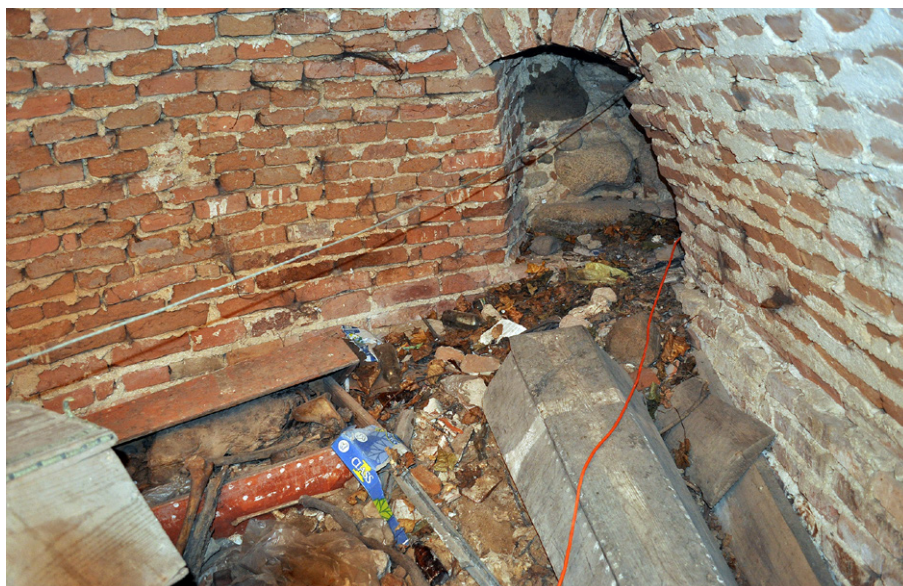
Fig. 7. Szczuczyn, Grajewo district, podlaskie voivodeship. View of the ventilation hole in the crypt under the Church of the Name of the Blessed Virgin Mary; state before the cleaning works were carried out (photo by A. Wojciechowska)
