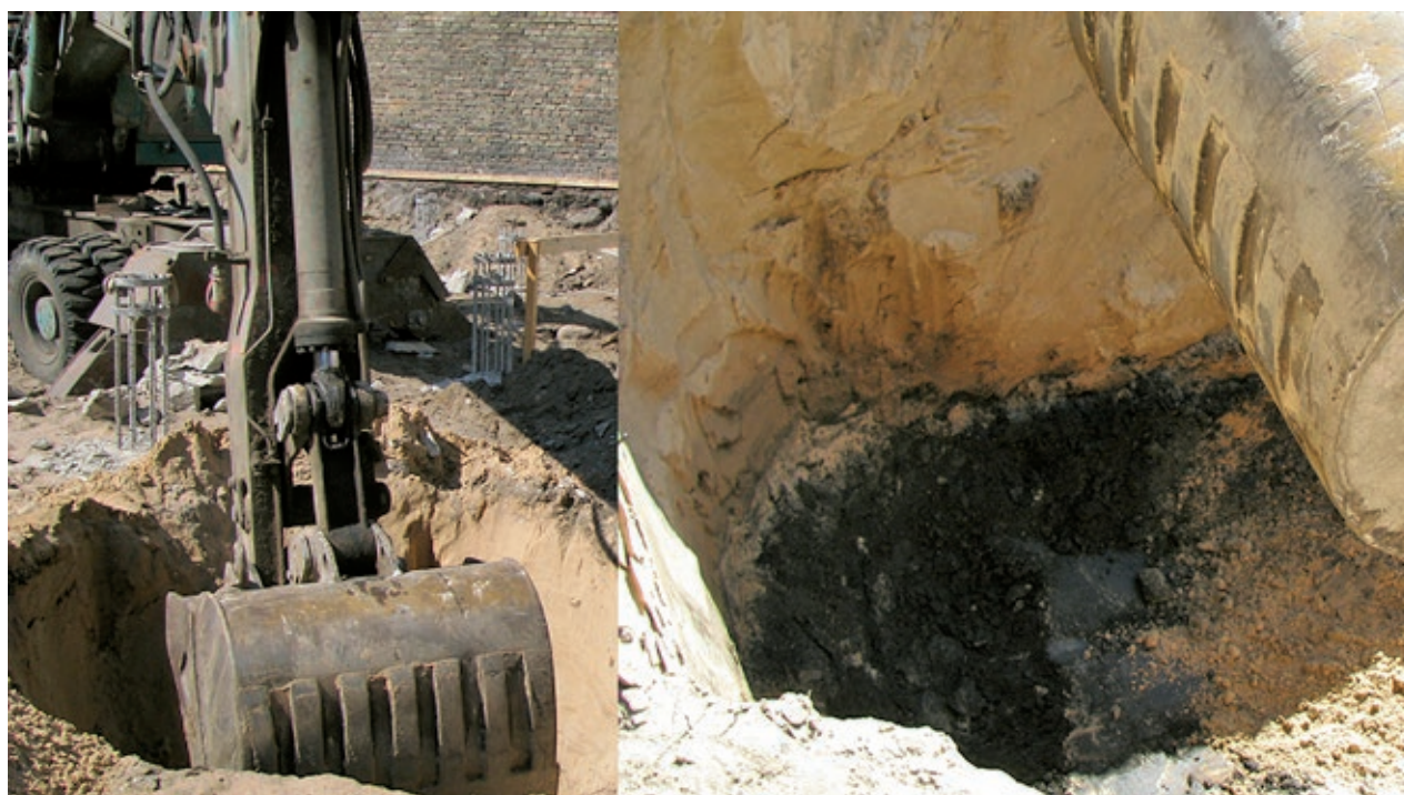
Fig. 10. Probing of subsoil-like sand layer (1.30-1.50m) and 14th-16th century cultural layer underneath them, Maiznieku Street, Ventspils, 2009 (Photo by Armands Vijups)
